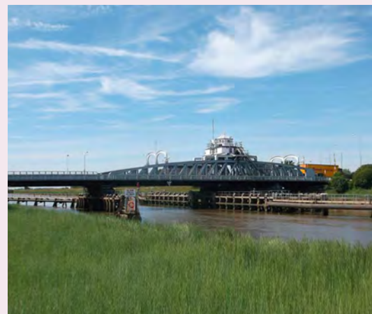
Cross Keys Bridge, Sutton Bridge
