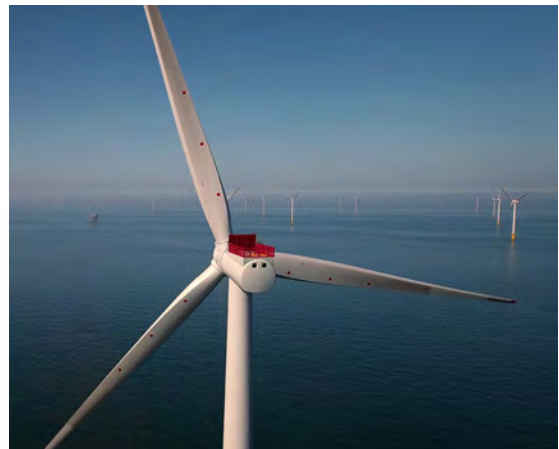
Offshore Wind Farm – Ørsted
