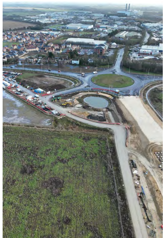
Spalding Western Relief Road in development – February 2023
